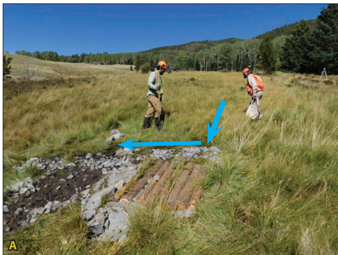
Figure 4.15A. In East Holman Creek, an incised channel with high and dry banks was mechanically collapsed to form a modified channel, which was armored with cobbles and integrated with down-gradient stabilization and flow-spreading structures. Figure 4.15B. In June of the following year, the structure was functioning properly to spread sheetflow to the former wetland on valley right. Blue arrows indicate flow path.
