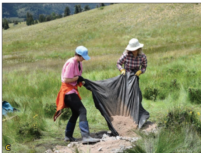
Figure 4.5A. In the photograph, wetland Carex grows through a log mat. Blue arrow indicates flow path. Figure 4.5B. In the photograph, base course materials are used to key structures together. Base course remains on the wetland surface after the structure is complete. Figure 4.5C. Geotextile fabric is used to deliver finer materials to stabilize a media luna with no impact to the surrounding wetland vegetation.
