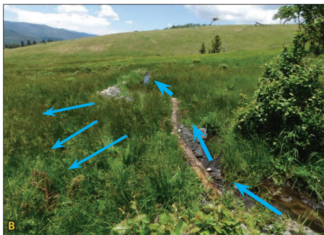
Figure 4.11A. The constructed keypoint diverts water from the channelized source via a lead-out berm to a reinforced spreader swale, sheetflow spreading structure, and stable return. Figure 4.11B. Photograph shows sheetflow below a stable return. Blue arrows indicate flow path.
