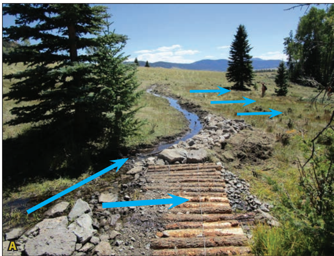
Figure 4.7A. A log step fall in West Holman Creek, serving as a flow splitter, stabilizes a head cut and splits water flow into an armored lead-out channel to a reinforced spreader swale, while allowing some flow to remain in the current channel to support downstream wetland vegetation. The log step fall is the constructed keypoint. Figure 4.7B. After one year, the swale is allowing water to both infiltrate below the berm and spill past a stable return at the end of the berm to rewet former wetland. Figure 4.7C. In the photograph, sheetflow from the lead-out swale and berm is visible travelling downvalley past the large and seedling conifers visible in both pictures (white arrows). Blue arrows indicate flow path.
