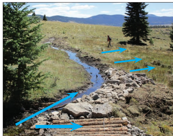
Figure 4.9. A rock armored lead-out berm and excavated channel split flows into a log reinforced spreader swale in the West Holman Creek drainage. Blue arrows indicate flow path.
