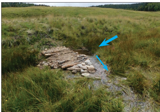
Figure 4.2. This log and rock flow splitter is built higher on the upstream side to spill water out of the incised channel and back onto the wetland surface. Blue arrows indicate flow path.
