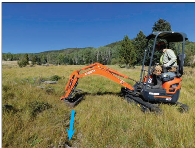
Figure 4.13. An incised channel bisecting this slope wetland complex in East Holman Creek has lowered the localized water table and caused the bank vegetation to dry out, leaving the channel vulnerable to further degradation. The channel is being stabilized by using a mini-excavator to collapse the high banks in order to raise the grade. Blue arrow indicates flow path.
