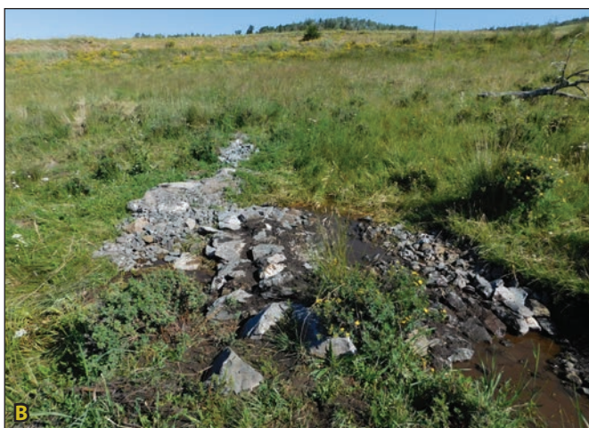
Figure 4.19A. A rock flow splitter was constructed in this incised channel to send water concentrated by an up-gradient culvert into an abandoned stock pond. Blue arrows indicate flow path. Figure 4.19B. Adaptive management to raise the elevation of the flow splitter (larger rocks) was necessary the year after the splitter was installed so that it could perform as intended.
