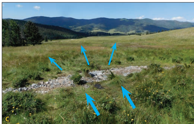
Figure 4.12A. Rock armor and excavated sod are used to create a lead-out berm to feed a reinforced spreader swale in East Holman Creek. Figure 4.12B. The water flows to the end of the berm. Figure 4.12C. Outflow from the berm is spread again with a rock media luna. Blue arrows indicate flow path.
