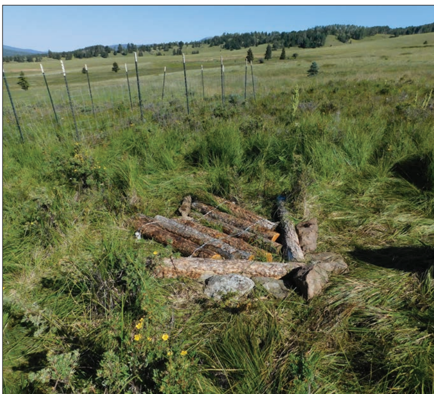
The above photograph shows a log mat flow splitter constructed to intercept channelized flow and convert it to sheetflow which will be intercepted by vegetation in the enclosure. Keyline Design principles lend themselves to linked treatment structures to maximize water spreading and harvesting benefits.
