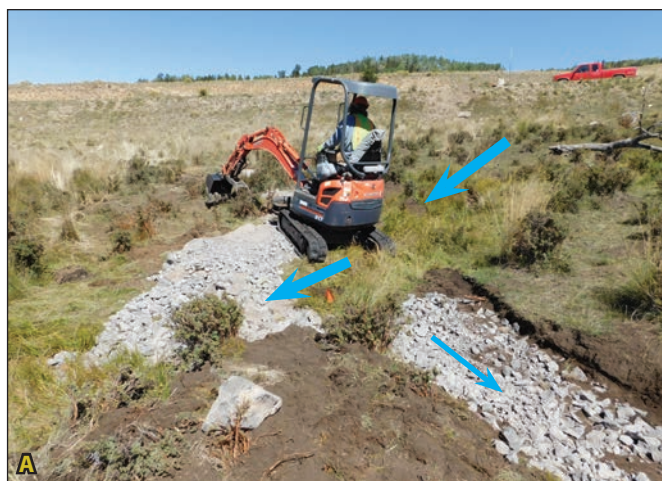
Figure 4.19A. A rock flow splitter was constructed in this incised channel to send water concentrated by an up-gradient culvert into an abandoned stock pond. Blue arrows indicate flow path. Figure 4.19B. Adaptive management to raise the elevation of the flow splitter (larger rocks) was necessary the year after the splitter was installed so that it could perform as intended.
