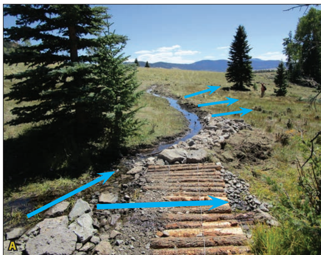
Figure 3.10A. The treatment train consists of a log mat flow splitter with a rock armored lead-out berm moving water into a swale with a log and sod reinforced berm. Figure 3.10B. The treatment train culminates in a stable return composed of two rock media lunas. Blue arrows indicate flow path.
