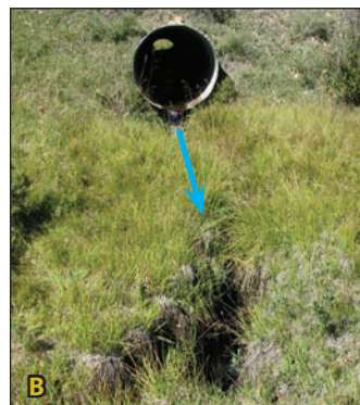
Figure 3.9A. Forest Service Road 1950 bisects the East Holman Creek. Figure 3.9B. A culvert concentrates flow, causing the channel to downcut below the culvert. Blue arrow indicates flow path. Figure 3.9C. An old stock pond interrupts sheetflow through the hillslope.
