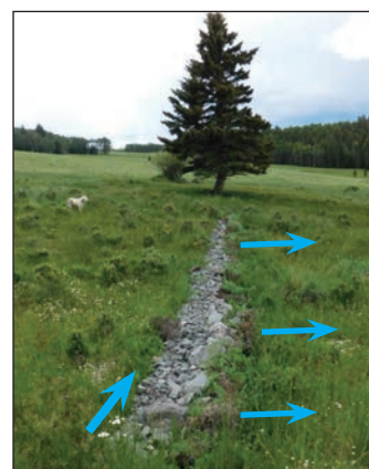
Figure 4.6. This swale was lined with angular cobble to increase stability because the wet meadow vegetation is currently not adequate to hold soil in a large flow event. Additional armoring is necessary until the swale has had some time to spread water and convert the wet meadow to wetland vegetation. Armoring also provides much needed protection from animal impacts, especially hoof shear. Blue arrows indicate flow path.
