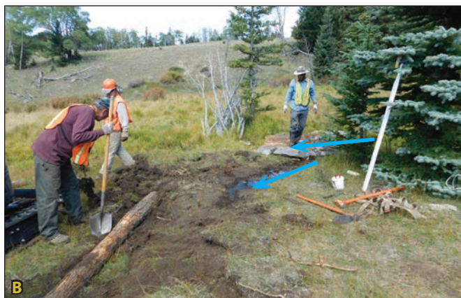
Figure 4.10A. The location for the log mat flow splitter was surveyed to ensure that water could be moved out of the channel at the proper elevation. Figure 4.10B. A swale was created to receive the water split from the channel by the log mat flow splitter. Figure 4.10C. The log structure delivers water to the swale. Figure 4.10D. A log mat is installed in the main channel below the flow splitter to raise the grade of the incised channel and further spread water over the wetland surface. Blue arrows indicate flow path.
