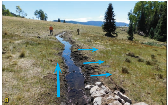
Figure 3.14A. The presence of Juncus (brownish-green colored rush) in the otherwise upland vegetation indicated that it might be possible to return this area to wetland obligate vegetation with increased water infiltration to the soil. Figure 3.14B. The photograph shows a constructed swale and berm at the end of a lead-out berm which moves water to the farthest extend possible. The treatment will increase water infiltration downvalley. Blue arrows indicate flow path.
