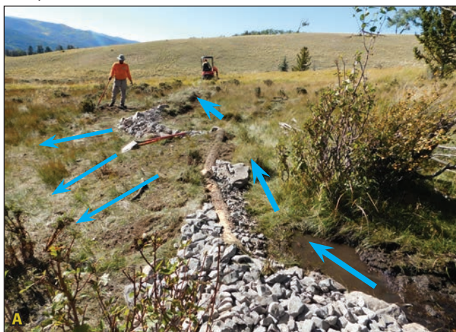
Figure 4.11A. The constructed keypoint diverts water from the channelized source via a lead-out berm to a reinforced spreader swale, sheetflow spreading structure, and stable return. Figure 4.11B. Photograph shows sheetflow below a stable return. Blue arrows indicate flow path.
