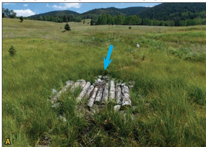
Figure 4.5A. In the photograph, wetland Carex grows through a log mat. Blue arrow indicates flow path. Figure 4.5B. In the photograph, base course materials are used to key structures together. Base course remains on the wetland surface after the structure is complete. Figure 4.5C. Geotextile fabric is used to deliver finer materials to stabilize a media luna with no impact to the surrounding wetland vegetation.
