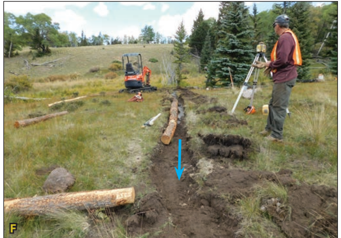
Figure 4.10E. A rock reinforced berm keeps the water in the swale. Figure 4.10F. Logs were buried in the downvalley edge of the swale to create a slightly higher berm. Blue arrows indicate flow path.
