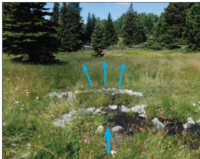
Figure 3.10A. The treatment train consists of a log mat flow splitter with a rock armored lead-out berm moving water into a swale with a log and sod reinforced berm. Figure 3.10B. The treatment train culminates in a stable return composed of two rock media lunas. Blue arrows indicate flow path.
