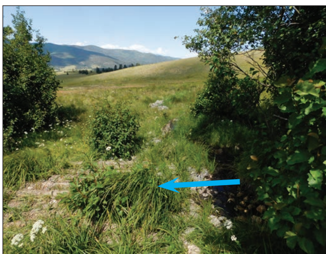
Figure 4.3. This log mat flow splitter was built upstream of a large headcut. It spreads the majority of flow to valley right through a rock and log reinforced lead-out berm. Existing vegetation was carefully incorporated into the flow splitting structure and new vegetation is colonizing the treatment area. The downstream area is kept saturated but the flow splitter prevents it from receiving erosive flows. Blue arrow indicates flow path.
