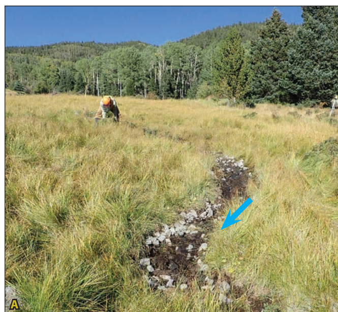
Figure 4.14A. The modified channel was stabilized with rock armor and one rock dams were installed as needed to further stabilize and aggrade the channel while spreading flows back onto the wetland surface. Figure 4.14B. The channel remained stable and sheetflow was re-established during snowmelt the following year, restoring floodplain connectivity. Blue arrows indicate flow path.
