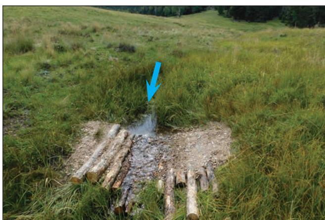
Figure 4.3. This log mat flow splitter was built upstream of a large headcut. It spreads the majority of flow to valley right through a rock and log reinforced lead-out berm. Existing vegetation was carefully incorporated into the flow splitting structure and new vegetation is colonizing the treatment area. The downstream area is kept saturated but the flow splitter prevents it from receiving erosive flows. Blue arrow indicates flow path.
