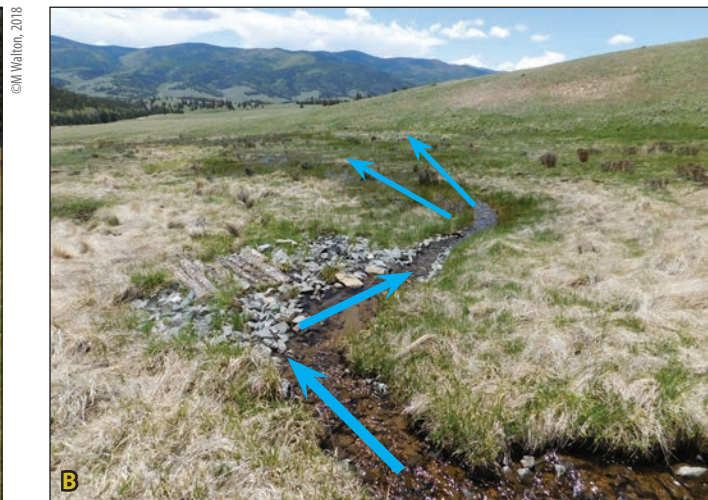
Figure 4.15A. In East Holman Creek, an incised channel with high and dry banks was mechanically collapsed to form a modified channel, which was armored with cobbles and integrated with down-gradient stabilization and flow-spreading structures. Figure 4.15B. In June of the following year, the structure was functioning properly to spread sheetflow to the former wetland on valley right. Blue arrows indicate flow path.
