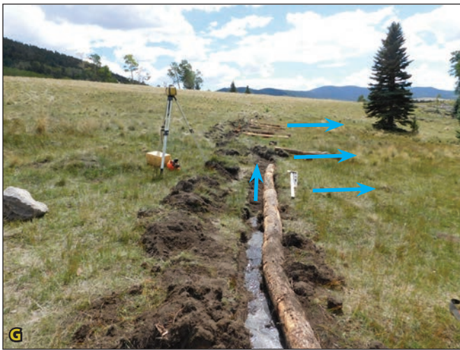
Figure 4.10G. Elevations were surveyed so that the swale was not at too steep an angle on the hillslope, which would have caused erosion. This also created a swale that followed the natural topography and not a straight line across the slope. Blue arrows indicate flow path. Figure 4.10H. The logs were keyed into the soil surface to minimize piping underneath and covered with sod.
