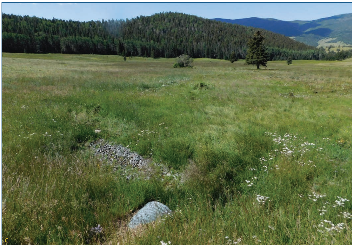
Figure 4.20A. The photograph shows sediment deposition from a culvert constricted flow path over an alluvial fan. Figure 4.20B. The sediment deposit was removed and a reinforced spreader swale was installed to convert concentrated outflow from the culvert into sheetflow over a greater area. Blue arrows indicate flow path. Figure 4.20C. After one good water year, the restored sheetflow into the wider area resulted in more productive vegetation.
