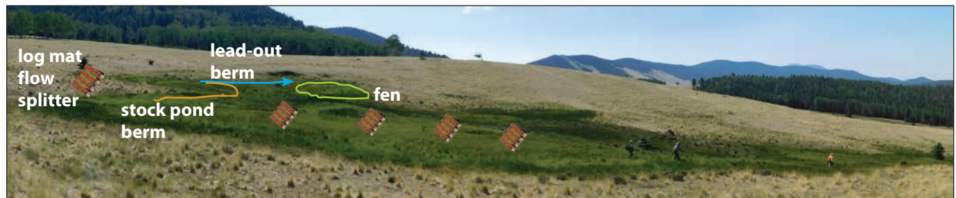
Figure 3.13. A treatment train on Middle Holman Creek continually spreads water from the main channel to wetland surfaces. Blue arrow indicates flow path.
