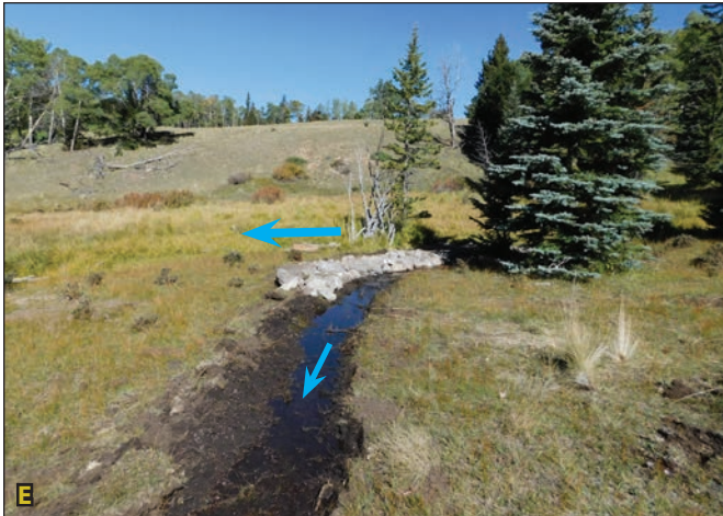
Figure 4.10E. A rock reinforced berm keeps the water in the swale. Figure 4.10F. Logs were buried in the downvalley edge of the swale to create a slightly higher berm. Blue arrows indicate flow path.
