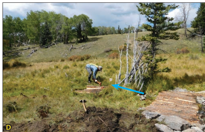
Figure 4.10A. The location for the log mat flow splitter was surveyed to ensure that water could be moved out of the channel at the proper elevation. Figure 4.10B. A swale was created to receive the water split from the channel by the log mat flow splitter. Figure 4.10C. The log structure delivers water to the swale. Figure 4.10D. A log mat is installed in the main channel below the flow splitter to raise the grade of the incised channel and further spread water over the wetland surface. Blue arrows indicate flow path.
